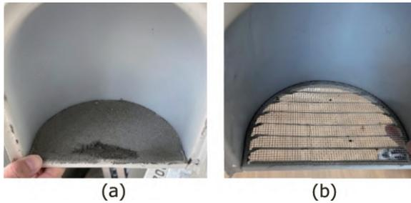
**Fig. 4:** Example before and after cleaning of louver panel of ventilation equipment. (a) Before cleaning (11m<sup>3</sup>/h). (b) After cleaning (176m<sup>3</sup>/h).
